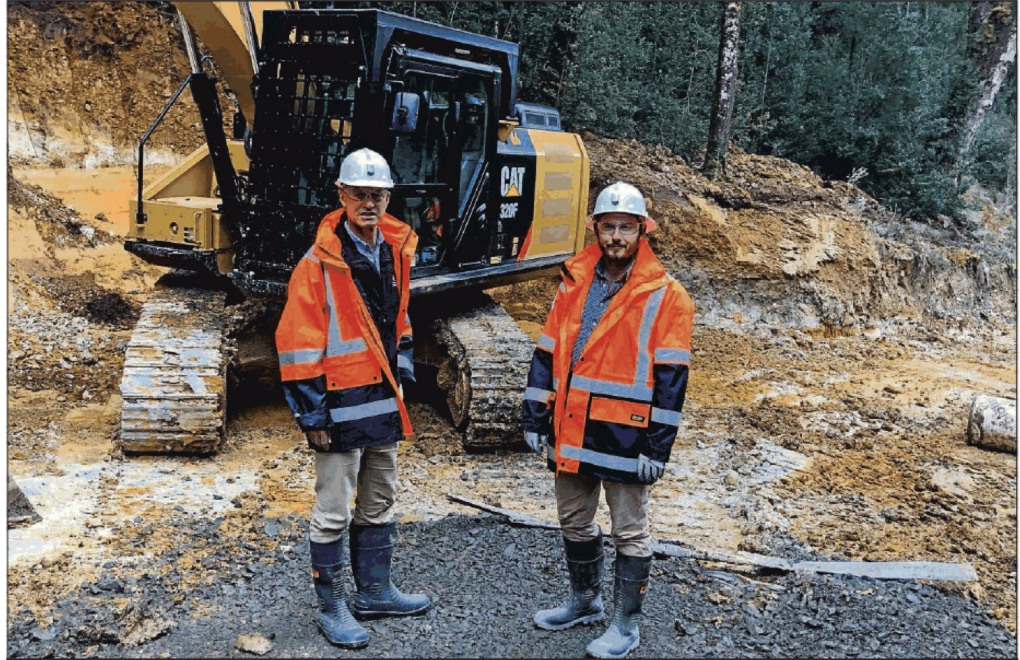
IN THE ZONE: Minister for Resources, Guy Barnett and Member for Braddon Felix Ellis on site at the proposed new tailings dam, a site which was earmarked for this purpose in 2014 by the Labor/Green government. Picture: Supplied
